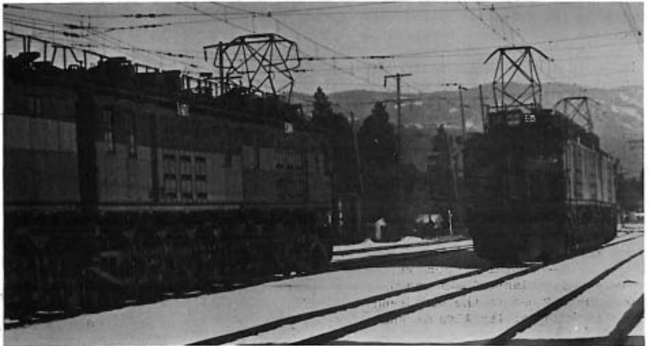
MILWAUKEE ROAD eastbound freight headed by E-50 (left) prepares to depart Cle Elum following arrival of E-25, running light, on 5 February 1971. Westbound E-25 had blown a transformer en route from Beverly to Boylston and left its train at Rye before limping on one unit to Cle Elum for temporary repairs.
