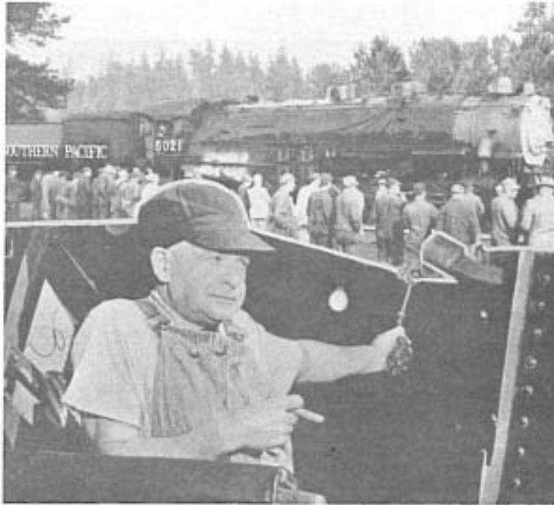
Last of her kind is Locomotive 5021, pictured as she was ready to pull out of the Portland area the morning of October 5, ending the employment of steam power on the northern part of our Portland Division. Inset shows Engineer A. B. Clancy, a veteran of 40 years with our railroad, as he tugged the whistle. With him were Ervin E. Schweiger, fireman, and Norman Park, brakeman.
