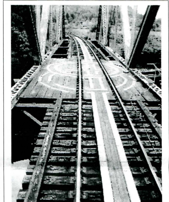
Ron McCoy contributed this photo of the walkways where the bridges are cranked.
