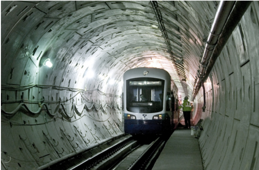
In the Beacon Hill Tunnel: A light rail car pushed by a special truck through the Beacon Hill Tunnel.
