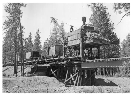
Above: A Brooks-Scanlon Lumber Company loco eases a string of log cars across a trestle in the pine country near Bend, Oregon. Left: It was moving day on Brooks-Scanlon when the photographer captured this view of a train with several skid shacks on log cars and a swing-boom McGiffert loader being pulled to a new location. *Photos, Jack Holst collection, PNWC-NRHS Archives*
