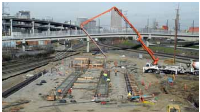
Below right: A concrete pump truck was used to deliver concrete to the forms. (March 11 photo by Chris Fussell)
