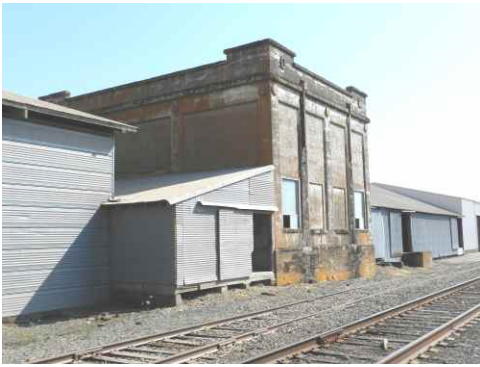
Substation at Cartney
