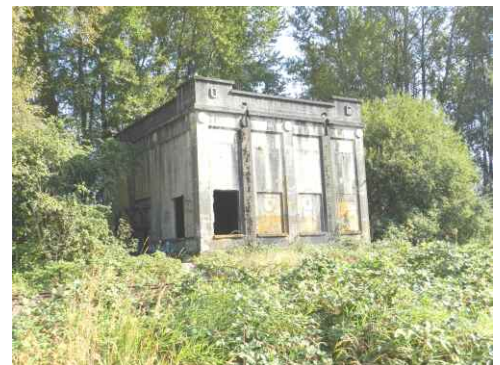
Substation at Pirtle
