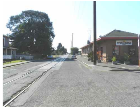
Junction City Station
