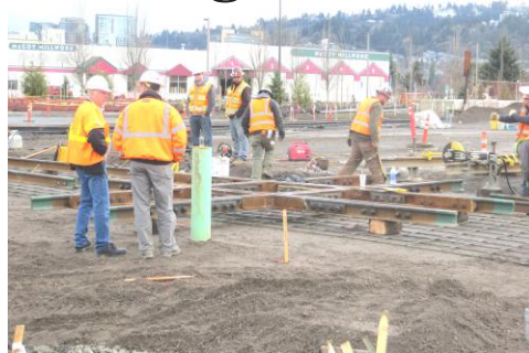
Dick Samuels inspecting the construction
