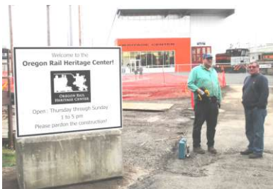
Construction continues around ORHC Activity being inspected by Keith Fleschner and Ed Immel
