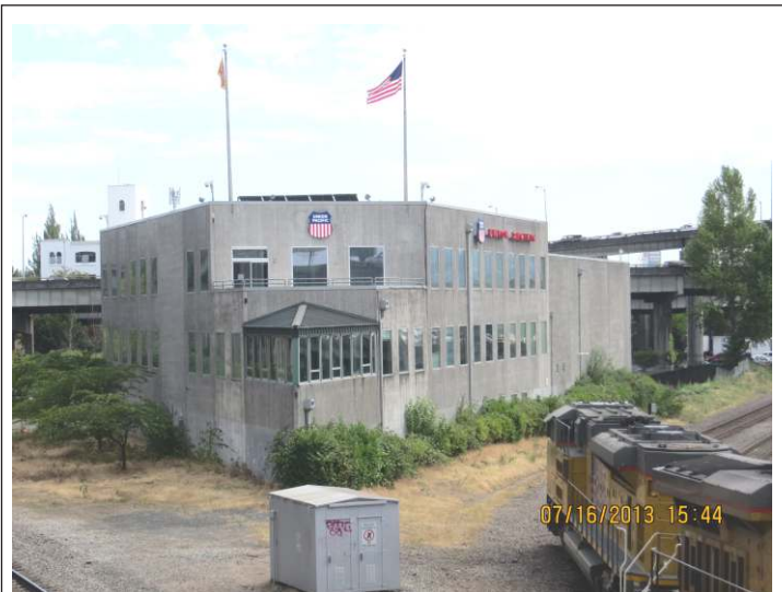
At the intersection of the Graham Line with the Brooklyn Sub-Division in NE Portland is the newly renovated Union Pacific Railroad office building now sporting the UP logo and flying the colors. A double-stack container train heads to the Brooklyn Intermodal yard; on the left, barely visible, is the Graham Line. Photo by Arlen Sheldrake.
