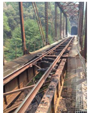
Siskiyou Line Bridge over the Middle Fork
