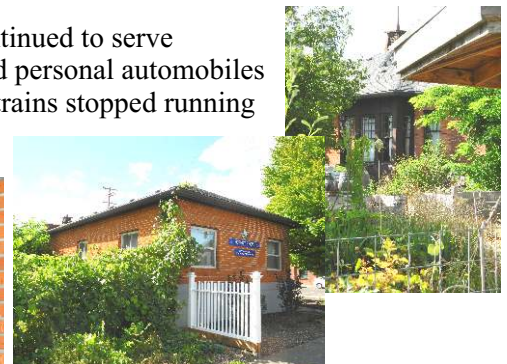
The roofline has changed over the years. The open area at the end (shown above) has been enclosed
