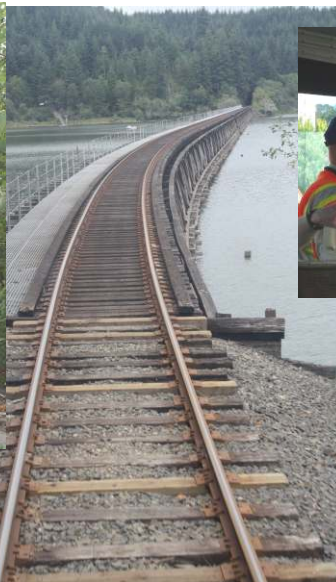
Coalbank Slough Bridge Built in 1914
