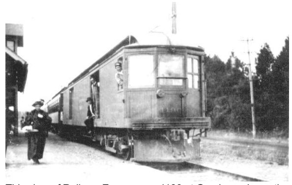
This view of Railway Express car 1190 at Gresham shows the newly added trolley pole in 1914. (Richard Thompson photo)
