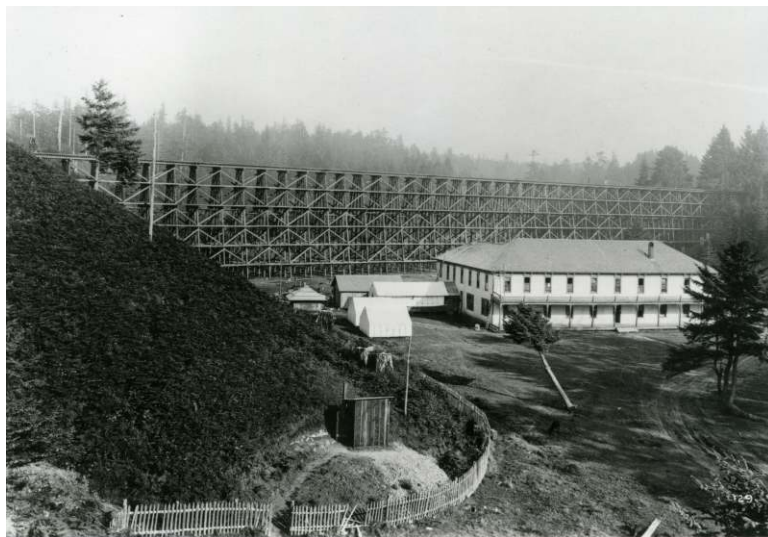
The Monterey Trestle, named for the hotel in the foreground, located just north Newport. Today a large fill on Hwy. 101 rests on the site. A.M. Prentiss photo No. 129
