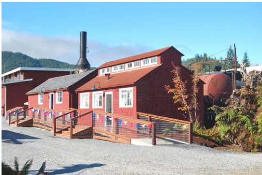
Some of the new buildings. One will feature a future theater.
