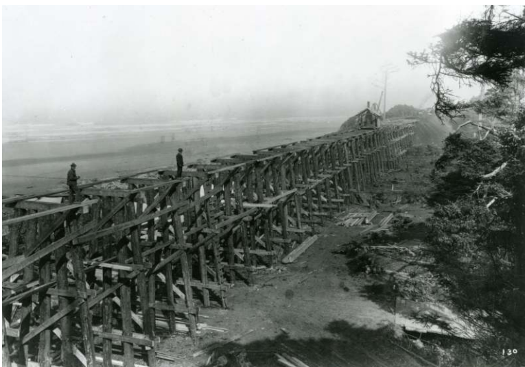
North of Newport the YN crossed numerous stream that required the building of several large trestles. Today's Hwy. 101 is atop the old grade. A.M. Prentiss photo No.130
