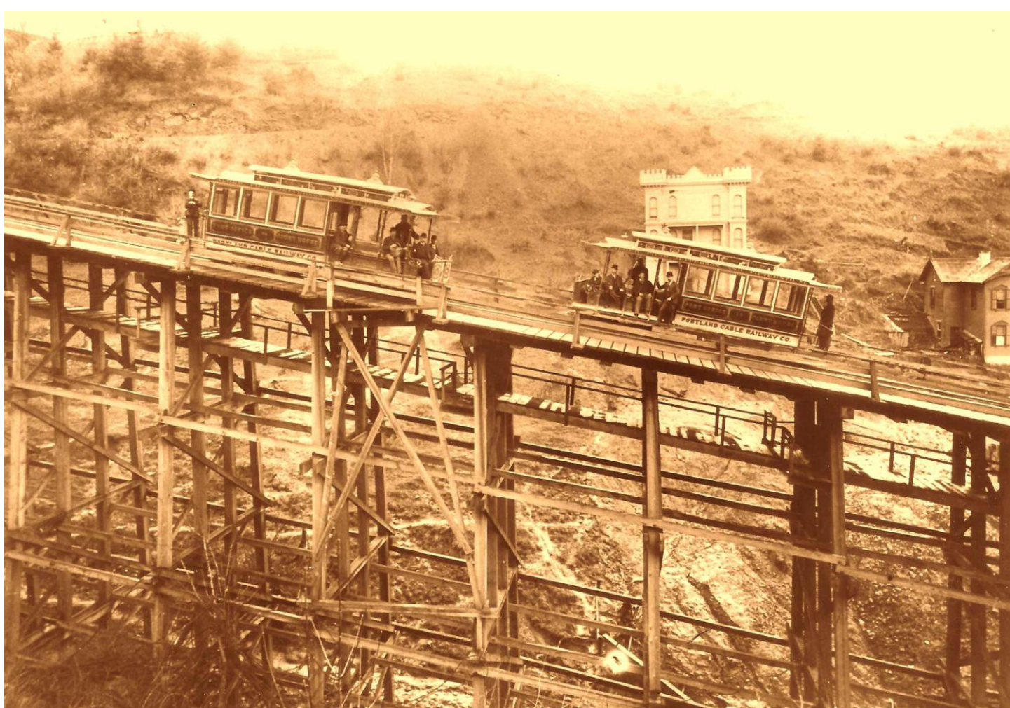
Two cable cars stopped on the trestle near Montgomery Drive. The house behind the car on the right is still there.
