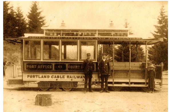
Cable car at the Spring Street turntable at the end of the line
