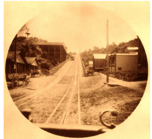
Taken from the back of a cable car, this photo shows the view up the trestle to Spring Street. The powerhouse and shops are to the right, out of view.
