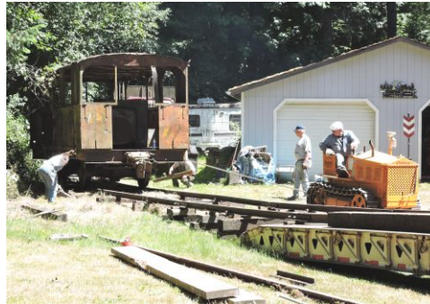
The Crew Speeder being Loaded
