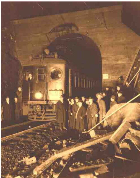
Allowing trains to bypass the dangerous Elk Rock Trestle, Elk Rock Tunnel opened December 5, 1921.
