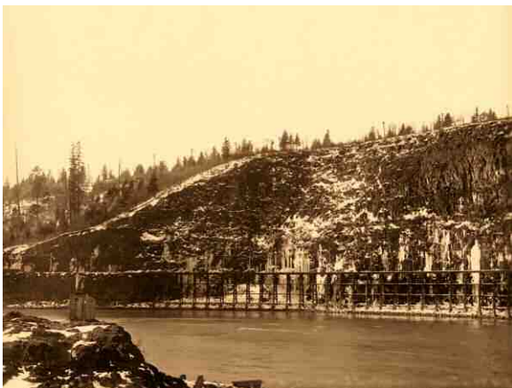
Frigid view of the 1400 foot Elk Rock Trestle on a snowy day, January 18, 1916.
