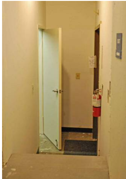
Receiving Hallway with new drywall.
