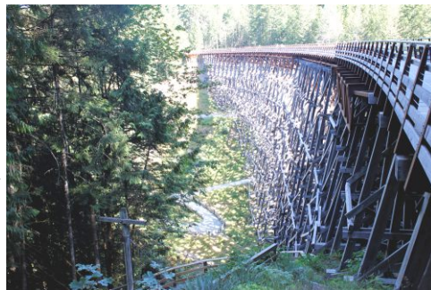
View of Restored Kinsol Trestle
