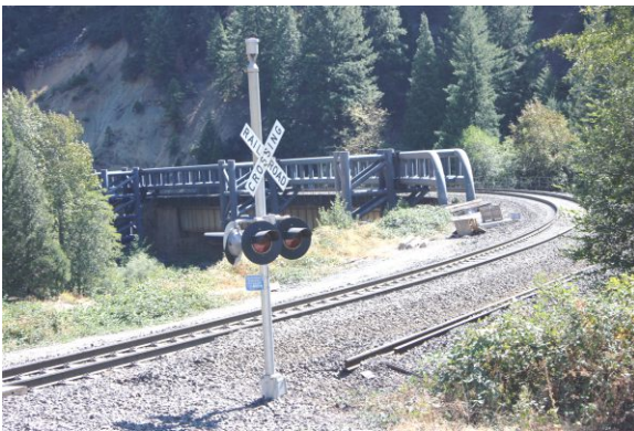
Cantara Loop Bridge
