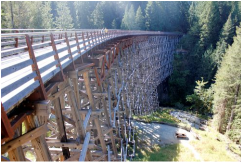
Another view of the Trestle
