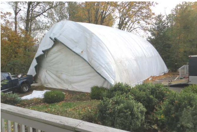
The all weather protection tent in October 2016
