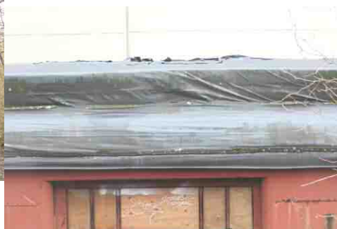
The Roof of Car No. 55
