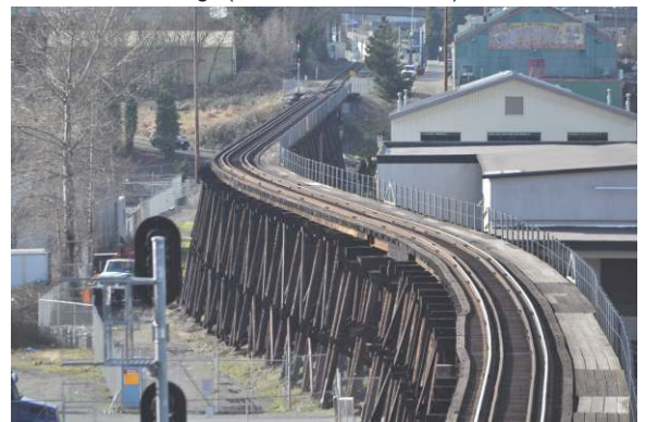
Milwaukee Road S-Turn timber trestle (above and below), built in 1908 and updated in 1937, is being replaced by a double track concrete bridge (shown at lower center).
