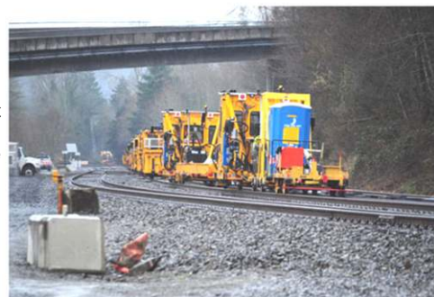
Tie replacement Crew moving through the Nisqually Valley.
