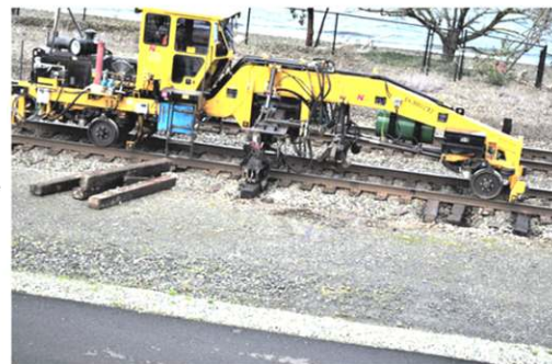
Inserting ties. Note: Removed ties are set aside and await pickup.
