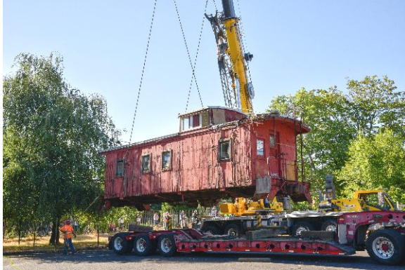
Caboose No. 507 being lifted into position (Photo by Jenna Wyatt)
