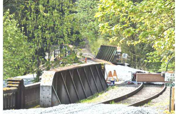
Closer view of the rail line bridge reconstruction
