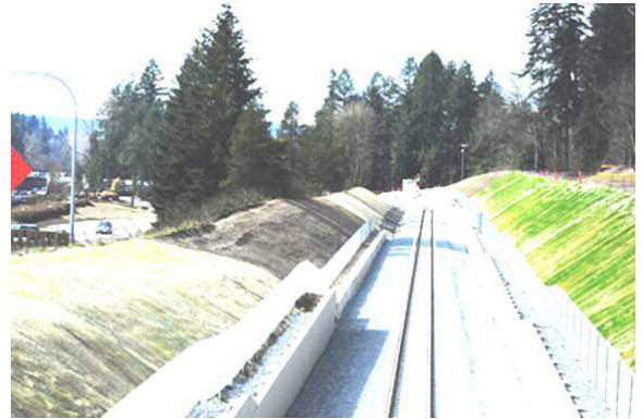
Looking west with new track, retaining walls and fence in place
