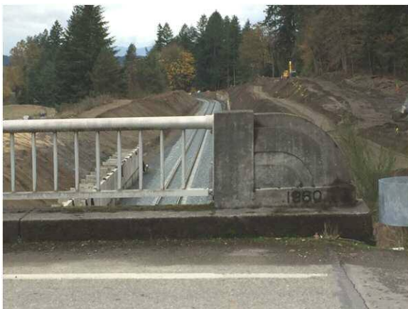
Picture from Mounts/Old Nisqually bridge west of DuPont. Bridge was built in 1960.
