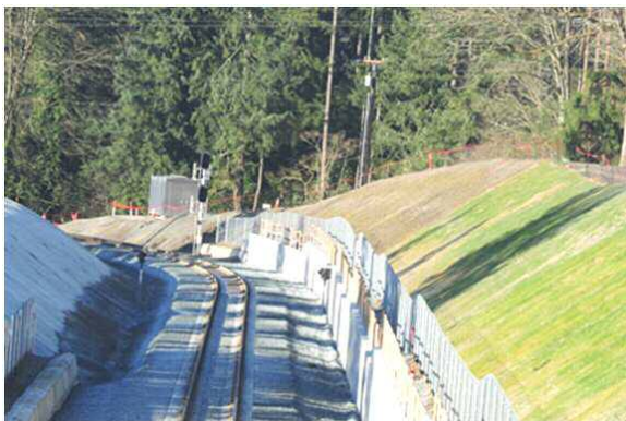
Track completed and just waiting for signal and clean up completion.
