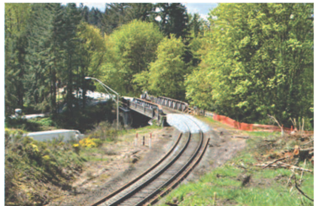
The I-5 bridge being refurbished
