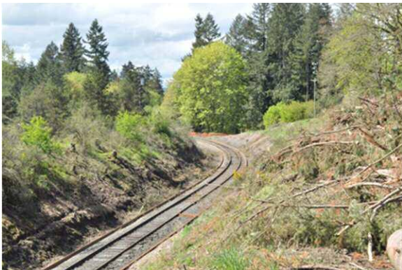
The Start of Construction
