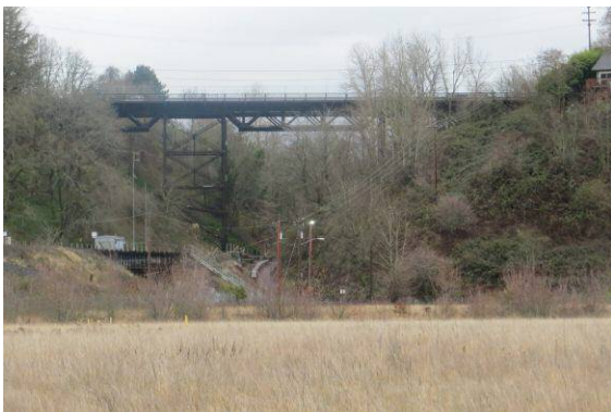
The Willamette Blvd. bridge & the West End of the Big Ditch
