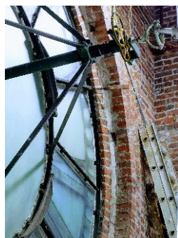
Detail of the Gearing behind the Clock Face
