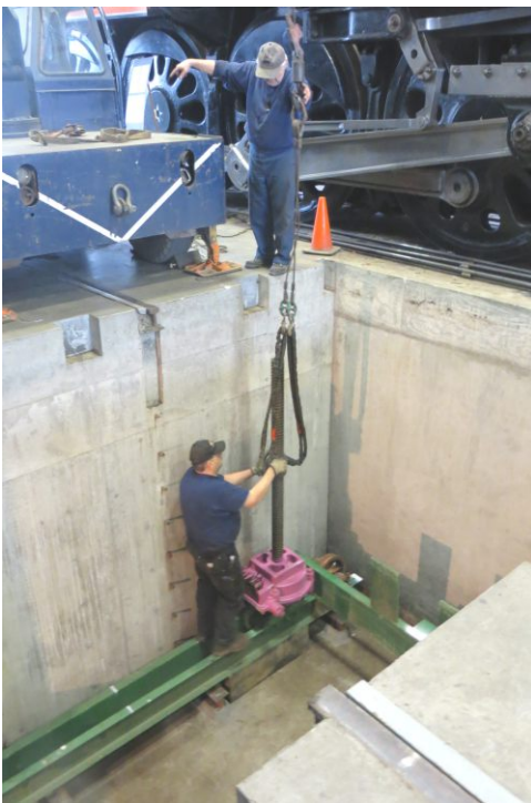
One of the Four Drop Table Screws being Installed
