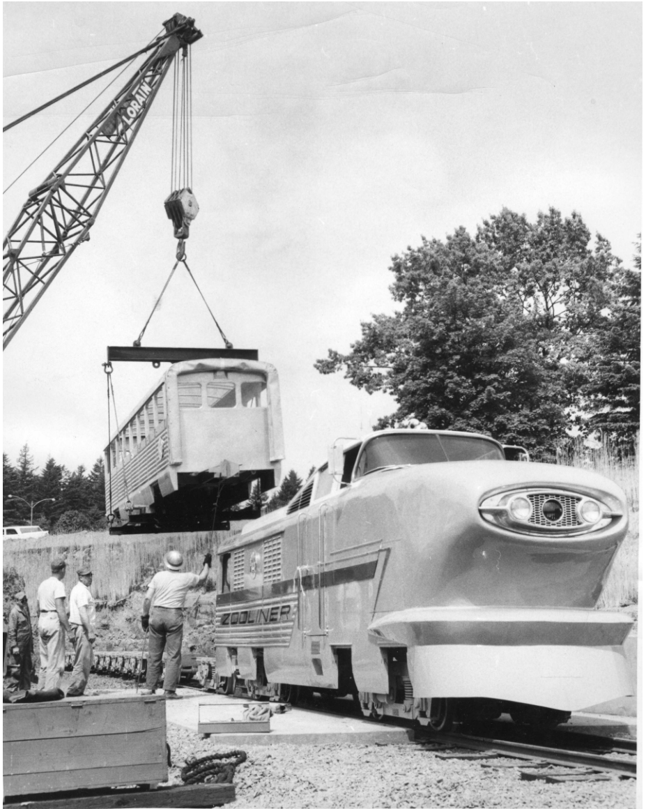
Delivery of the Zooliner to the new zoo railway. The locomotive is sitting over the service pit, still used today, adjacent to where the tunnel and shops would later be built.
