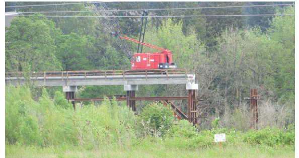
Photo of the Trestle Construction
