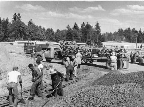
In May of 1958, crews are ballasting and tamping the new track where the train station would later be built. In the background is a flat-bed tractor-trailer truck from Northwest Marine Iron Works delivering the trucks (wheel sets) for the entire Zooliner train. Just beyond the tractor can be seen the “construction train.”
