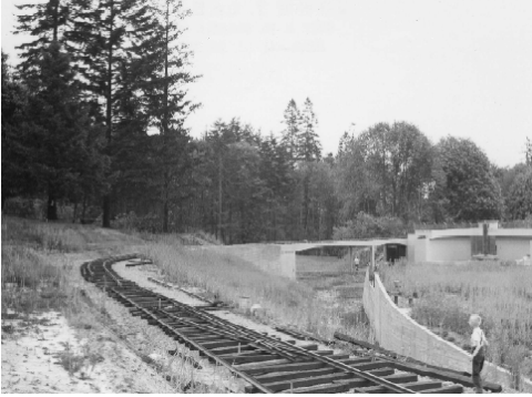
Laying the track in the spring of 1958
