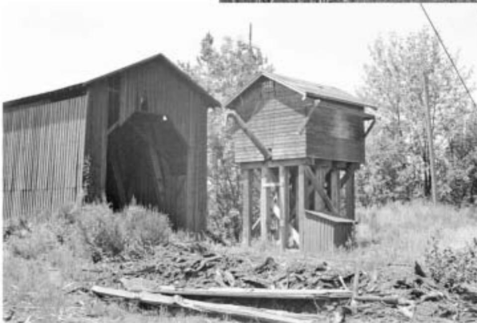
These three photos, taken in 1952 during the scrapping of the railroad, show the covered bridge as it appeared at the end of its working life. The siding was relatively intact, and the roofing was complete. The water tank was located to serve either the log dump track (left in lower photo) or the mainline. All photos, Ivan Ergish collection, Oso Publishing Company
