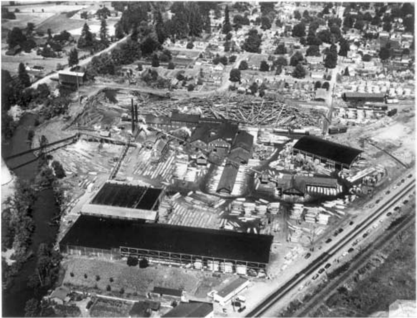
This air photo, probably taken in the late 1940s, shows the mill complex at its peak. Visible in the upper left corner is the covered bridge. In the middle left is the waste burner, connected to the mill by a conveyor that spans the river. The mill itself is in the center with the dry kilns and lumber storage below it. In the lower right are the tracks of the Southern Pacific and Highway 99. Photo, Casey Carlson collection, TimberTimes
