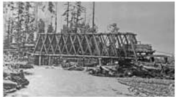
Two other railroad Howe trusses exist in the Northwest. Shown above is the Dungeness River span, located just west of Sequim, Washington. The photo on the left was taken just before it was removed from service in the mid-1980s. On the right is a photo taken during its construction in 1915. It is now the centerpiece of Railroad Bridge Park. Below are photos taken in 2002 of a partially covered Howe truss originally constructed for an interurban line that ran from Spokane to the Pullman area. The bridge is located near Colfax, Washington and is in private ownership. Photos, Hauff collection
