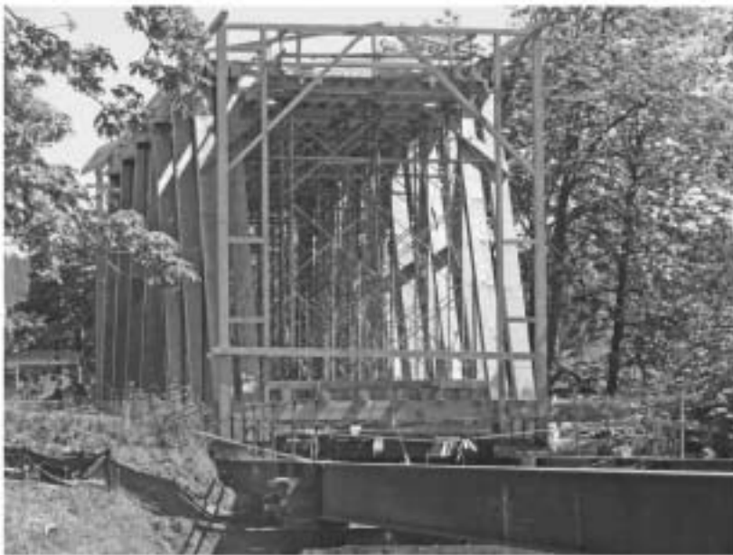
Above: Reconstruction of the bridge took place on the old railroad roadbed just east of the river. This eliminated any need to work over the water and allowed access to both the inside and outside of the trusses. In this photo, taken in July 2011, scaffolding has been erected to facilitate the installation of the upper cross-members and diagonals.
