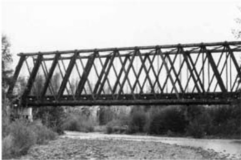
Two other railroad Howe trusses exist in the Northwest. Shown above is the Dungeness River span, located just west of Sequim, Washington. The photo on the left was taken just before it was removed from service in the mid-1980s. On the right is a photo taken during its construction in 1915. It is now the centerpiece of Railroad Bridge Park. Below are photos taken in 2002 of a partially covered Howe truss originally constructed for an interurban line that ran from Spokane to the Pullman area. The bridge is located near Colfax, Washington and is in private ownership. Photos, Hauff collection
